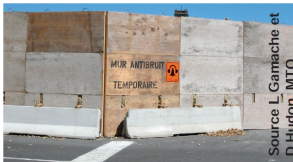
Plywood barriers with a soundproofing product limit nuisance in areas affected by medium- and long-term work. Source: Lafontaine et al. , p. 12 (42).
