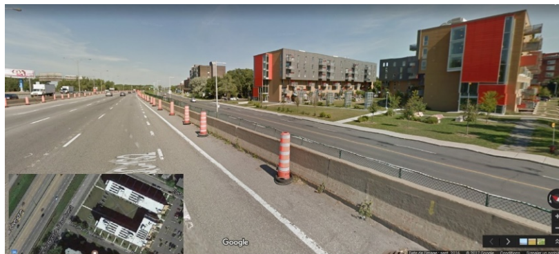
Photo 18 Example of a non-optimal shape design for a building exposed to road noise
