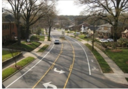
Transformation of an undivided, four-lane boulevard into a “complete street” (traffic flow: 20,000 vehicles/day) with a center turn lane, bike lanes and ramps for sidewalk access. City of Charlotte, Mecklenburg County (NC): East Boulevard. Photo credit: Charmcheck.org
