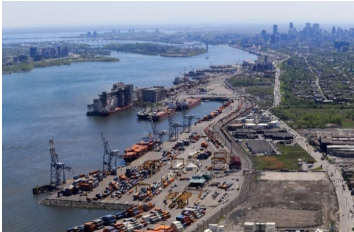
Aerial view of a part of the Port of Montréal.
