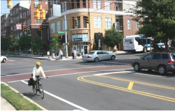
Downtown intersection with many features: highly visible pedestrian crosswalks, bike lanes, addition of trees and good pavement marking. City of Charlotte, Mecklenburg County (NC). Photo credit: City of Charlotte, Department of Transportation).
