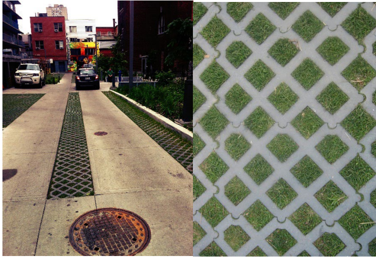
Figure 4 Slabs that allow for plant growth
